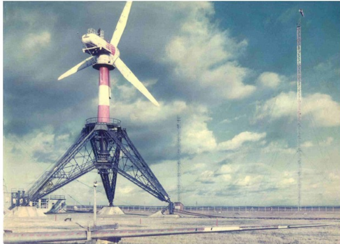
Neyrpic : 130kW - Ø21 (1962-66) & 1000 kW – Ø35 (63) Asynchronous generator + gearbox + Pitch regulation
